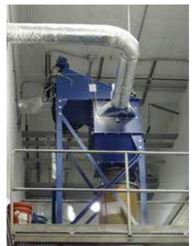
CPC-3 - Powdered milk dust in cheese factory 1,200 cfm (2,038 m 3 /h)
